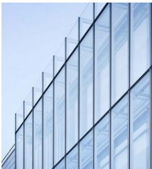
Curtain Wall with Insulated Glass
